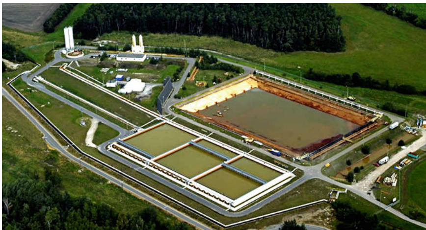
Fig. 4.10 Chemical treatment plant (Grubenwasserreinigungsanlage GWRA. Photo: P. Radke/LMBV) Rainitz, treating acidic filling water of the future Lake Ilse/Pit Meuro in the Lausatian lignite district, eastern Germany. The final capacity will be 3 \text{ m}^3/\text{s}
