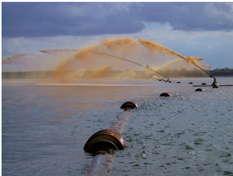
Fig. 4.3 Distribution of lime in Lake Koschen by floating pipeline and circular sprinklers (Photo: Egbert Gassert 2004)
