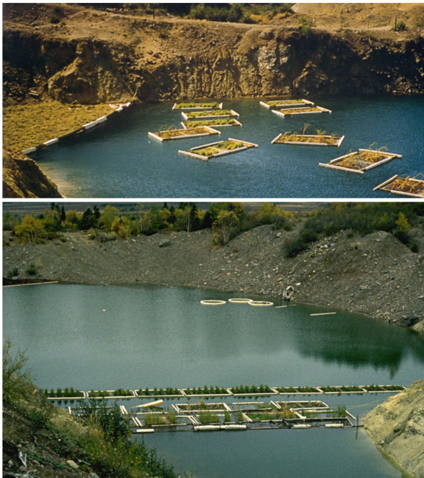
Fig. 5.63 a The acidic Oriental West Pit lake when peat and straw were added to form microbial active sediments. b Vegetation rafts to reduce wind circulation to the bottom of the pit
